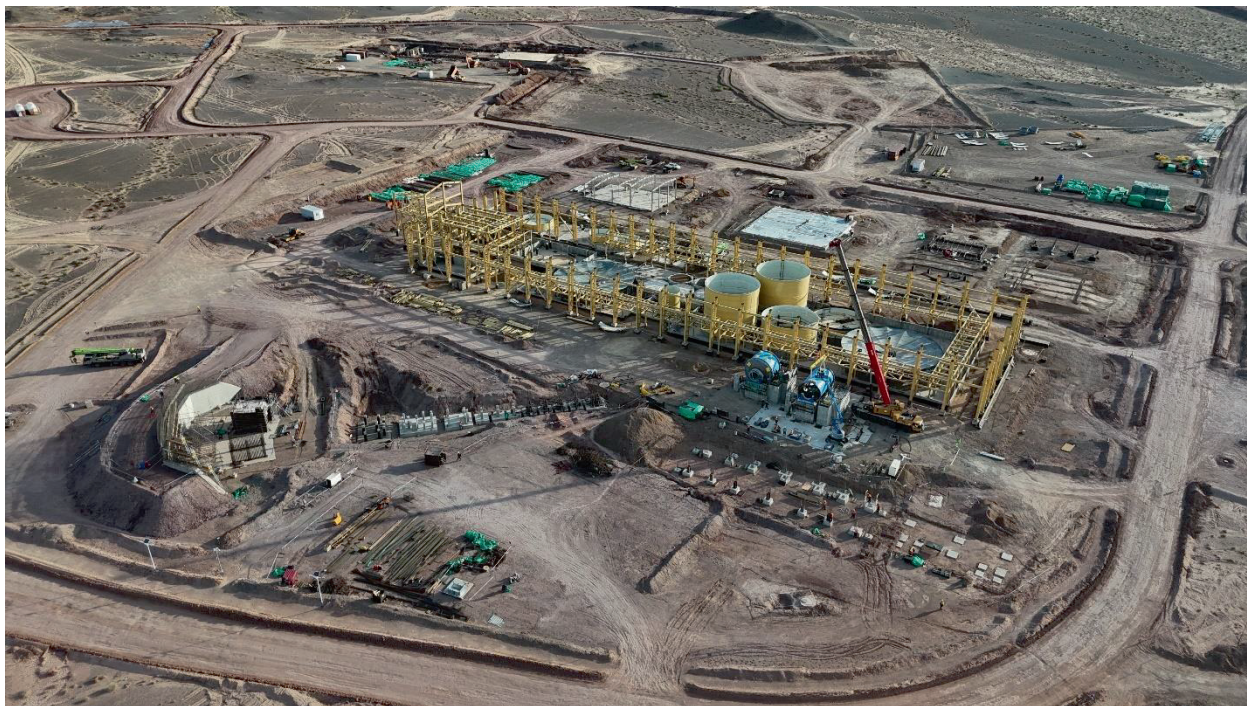
Photo: Processing plant construction at BKH mine as at 31 July 2024.
